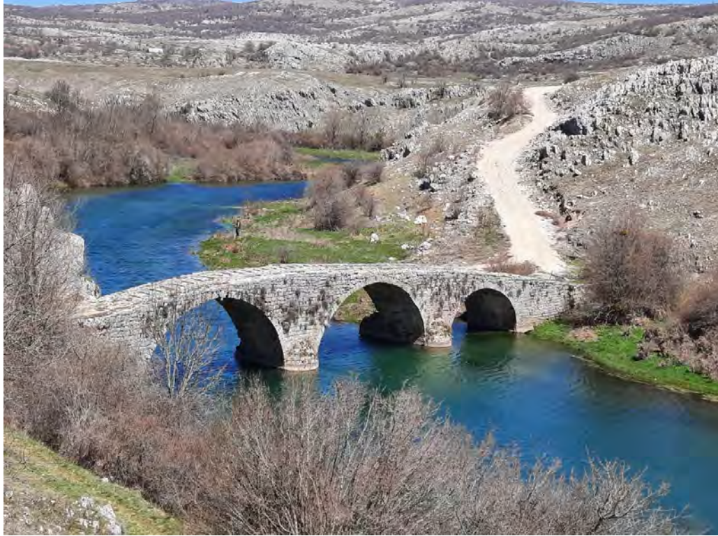
Photo 2.77 Ovčiji Brod Bridge, Zalomka River, Herzegovina. Natalija Samardžić
