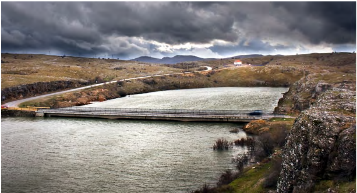
Photos 2.39 Gvozdeni Most Bridge, Zalomka River, Herzegovina. Željko Zubac
