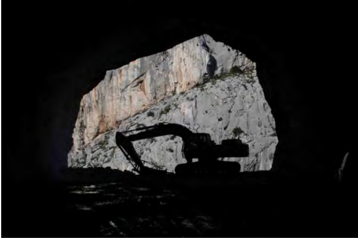
Photo 10.44 Omiš Tunnel, Croatia . Mladen Garašić
