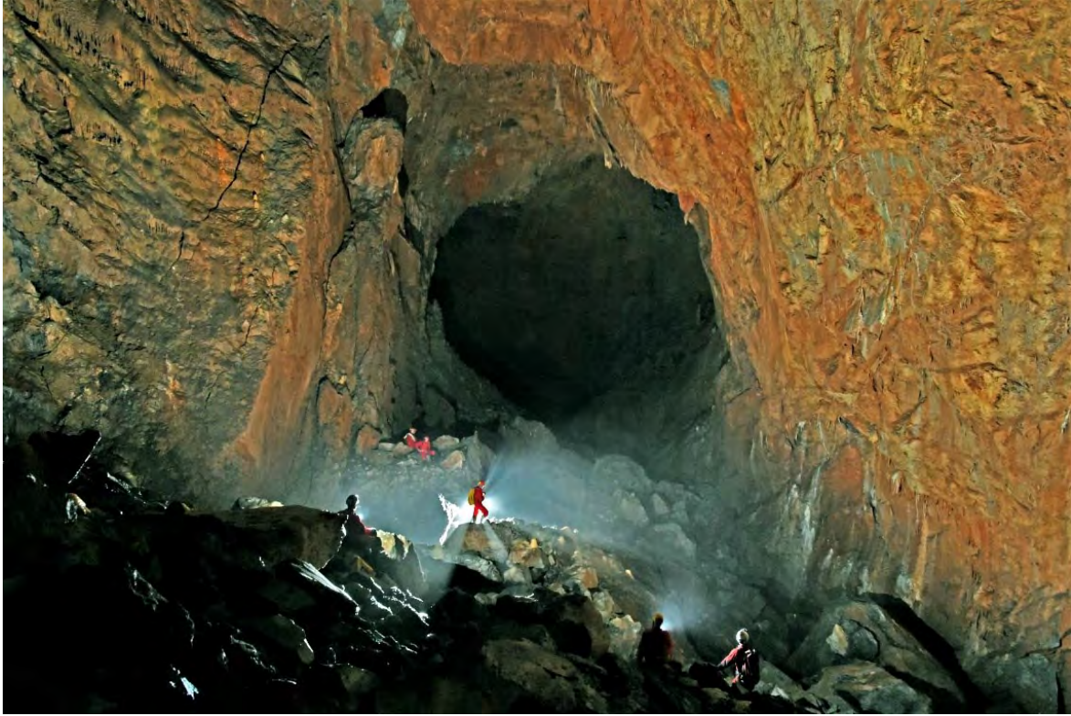
Photo 7.47 Cavern, Tunnel Construction, Highway A-1, Velebit Mt., Croatia. Mladen Garašić
