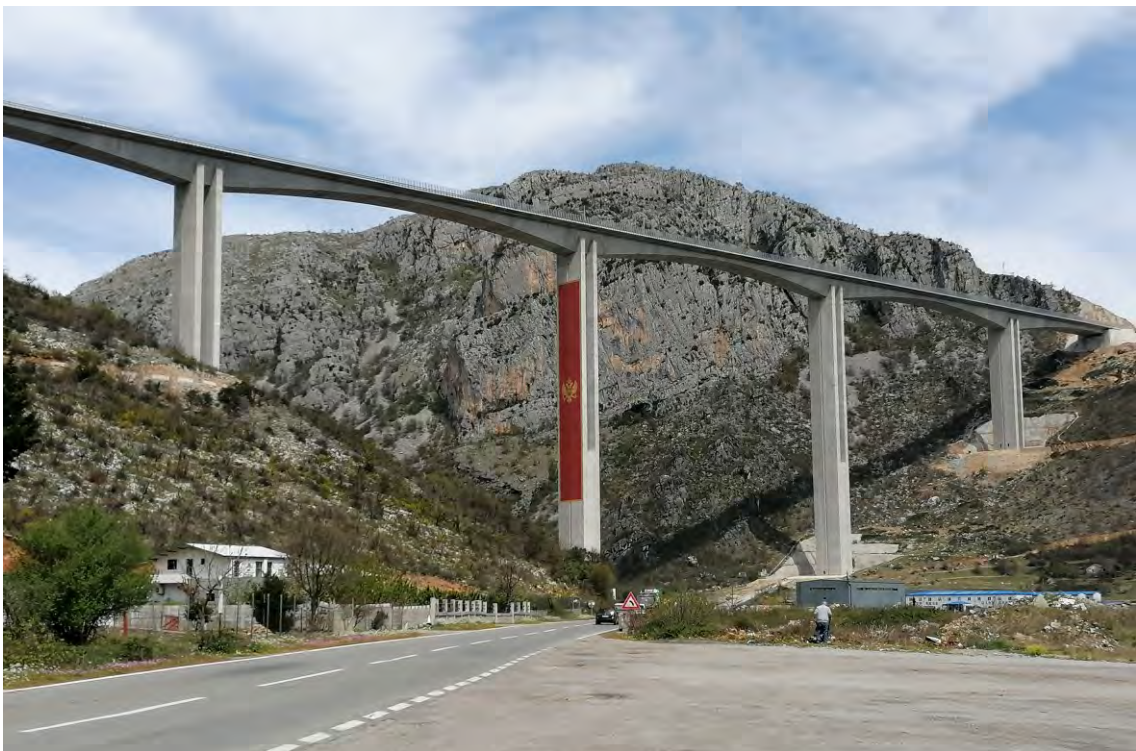
Photo 10.43 New Moračica Bridge, Montenegro. Zoran Stevanović
