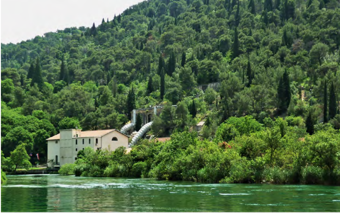
Photo 10.47 Jaruga Hydroelectric Plant, Krka River, Croatia. Neven Kresic
