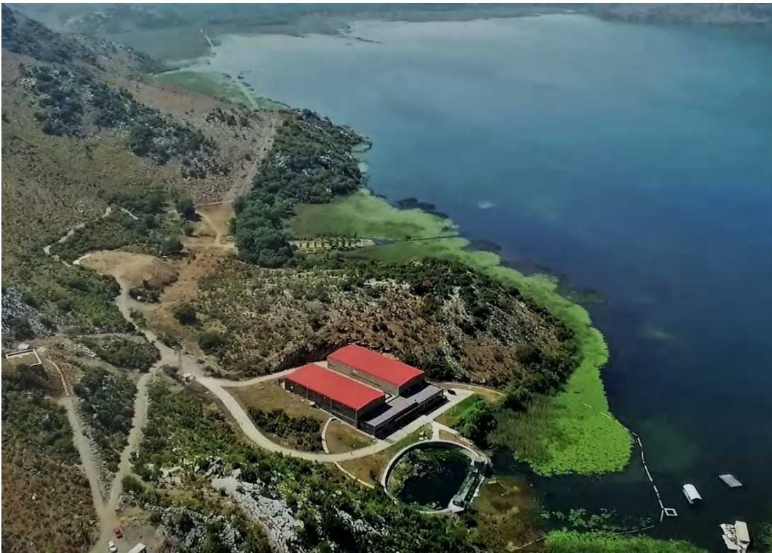
Photo 5.33 Bolje Sestre Spring . Courtesy of Regional Waterworks of Montenegro Coast
